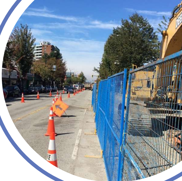
FortisBC's Traffic Management Approach
