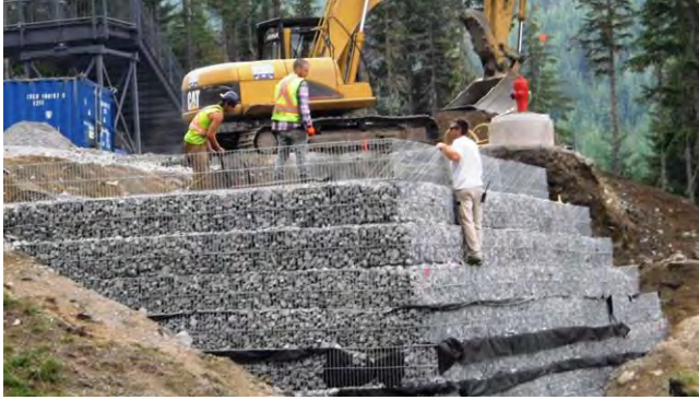
Photo 12: Example of a geogrid-reinforced SierraScape retaining wall under construction.
