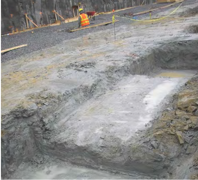
Photo 7: Example of a suitably prepared foundation subgrade.
