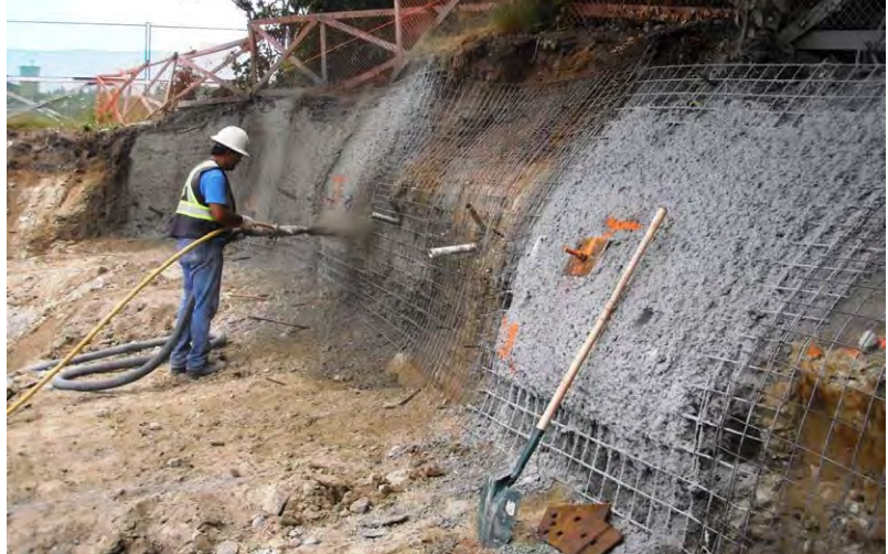
Photo 3: Installing temporary excavation shoring (shotcrete and anchors).
