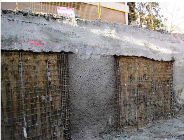
Photo 10: Example of a temporary shoring system comprising pipe piles that do not encroach onto neighbouring property.
