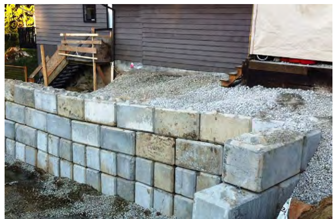
Photo 9: Example of a previously unsafe temporary excavation slope that has been stabilized with a Lock Block retaining wall.
