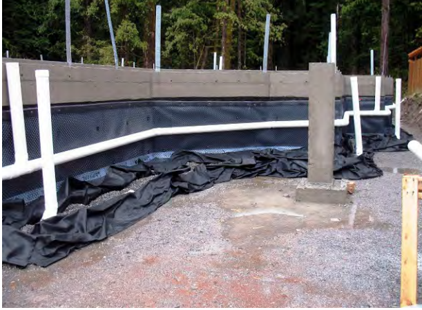
Photo 11: Example of a foundation wall with drainage membrane applied over the damp-proofing agent and PVC foundation drain pipe bedded in clear gravel wrapped in filter cloth.
