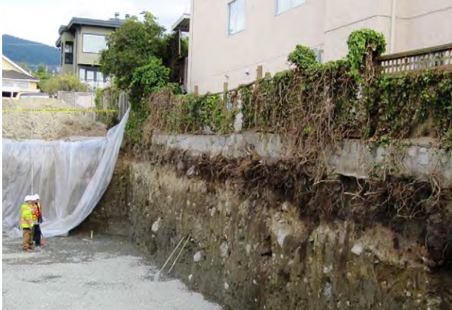
Photo 8: Example of an unsafe temporary excavation slope (unsupported).
